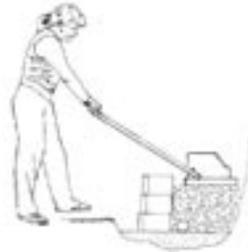
4. Level the gravel base from front to back and side to side. This procedure will ensure a straight and stable wall.
