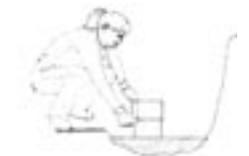
6. As you lay each unit of the first row, check the level of the block from side to side and front to back. Careful preparation of this base row is the key to having a successful and attractive finished project.
